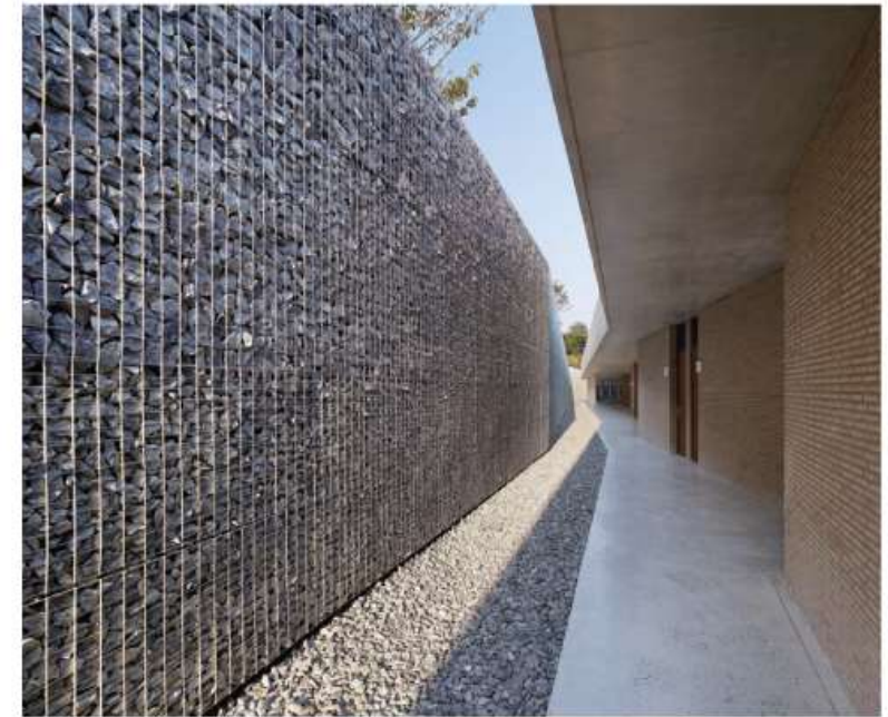
Outdoor corridor of the dormitory
