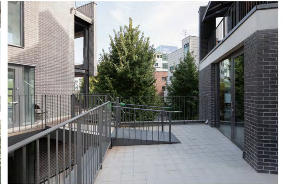
공사 도중 인접 대지를 매입하게 되어 현재의 1동과 2동의 수평적 연계가 더해졌다. Adjacent land was purchased during the construction stage, and the connection between the current first and second building was added.
