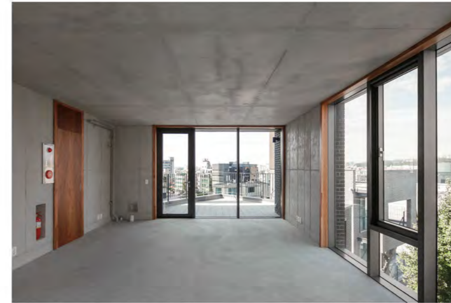
내부 공간은 유로폼노출콘크리트와 에폭시페인트의 중성적인 마감에 창틀에는 집성목합판을 추가하였다. The interior space was finished neutrally with a euro form exposed concrete and epoxy paint, and edge glued plywood panels were added onto the window frames.
